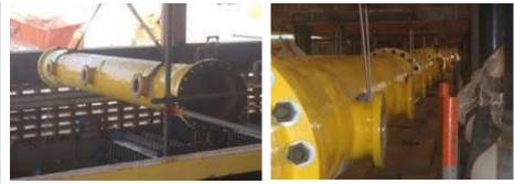
Contact Molded Fiberglass Pipes and Fittings for a Chlorine Processing Plant
