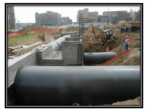
Pressure Application – FRP can be used for pressure applications, but thorough design analysis and consideration must be given to ensure adequate safety factors. Fiber-glass-reinforced pipe has been used for applications up to 1,200 psi. Large diameter (7 ft dia. x 17 ft high) vessels have been built for pressures up to 160 psi at 220° F. Even higher-pressure applications have been achieved in the military area with exotic reinforcement materials and epoxy resins.
